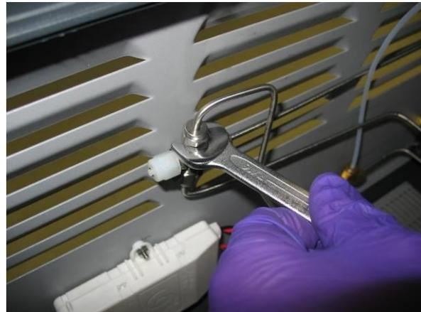
Figure 15 – installing the new quick connect.
